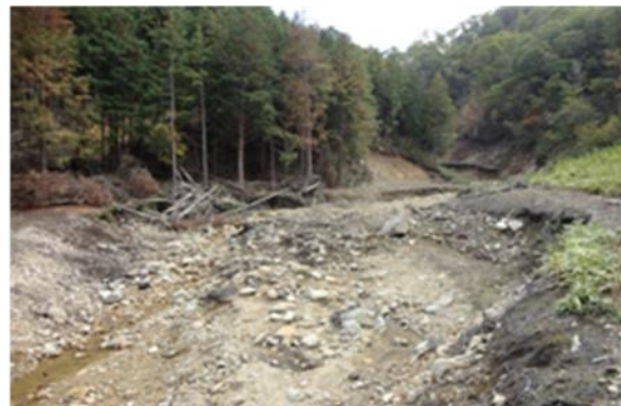
Fig 9: Upstream face of Site #5 showing tree stumps and cleared debris path
