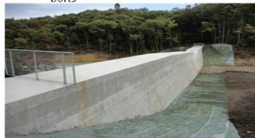
Fig 7: Check Dam at Site #5
