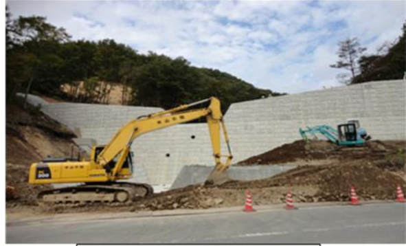
fig 2: Remediation work at Site #4
