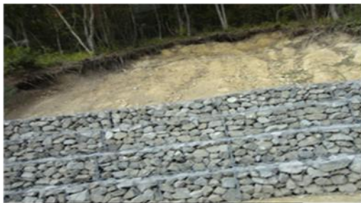
Fig 4: Gabion Walls at site #2
