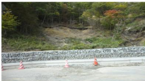
Fig 6: Gabion Walls at the Site #4
