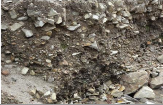
fig 1: Characteristic material composition at toe of landslide #5
